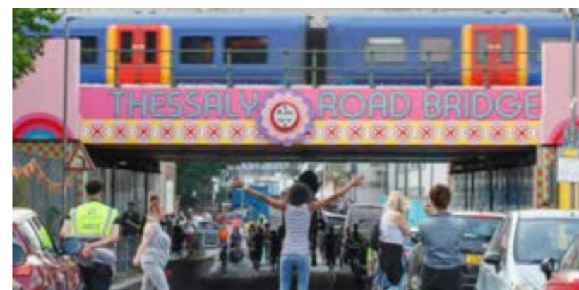
A colourful railway underpass upgrade for Thessaly Road Bridge. Credit: Yinka Llori
