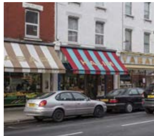
Shopfront and awning upgrades on Green Lanes, London. Credit: East Architecture
