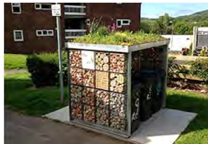
Bin enclosure with wildlife supporting features on its top and sides. Credit: Green Roof Shelters
