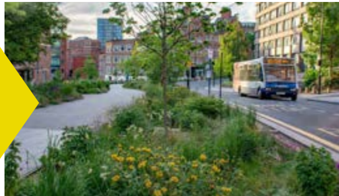
Precedent: Grey to Green, Sheffield. A transformative project to create greenery and improved active travel infrastructure.
